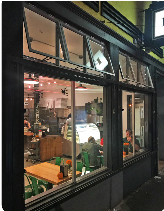
Operable transom windows address the pedestrian.
