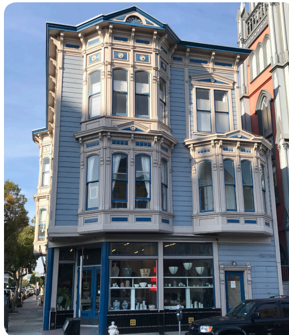
Victorian buildings provide a richness in ornamentation that is essential to Calle 24's character.
