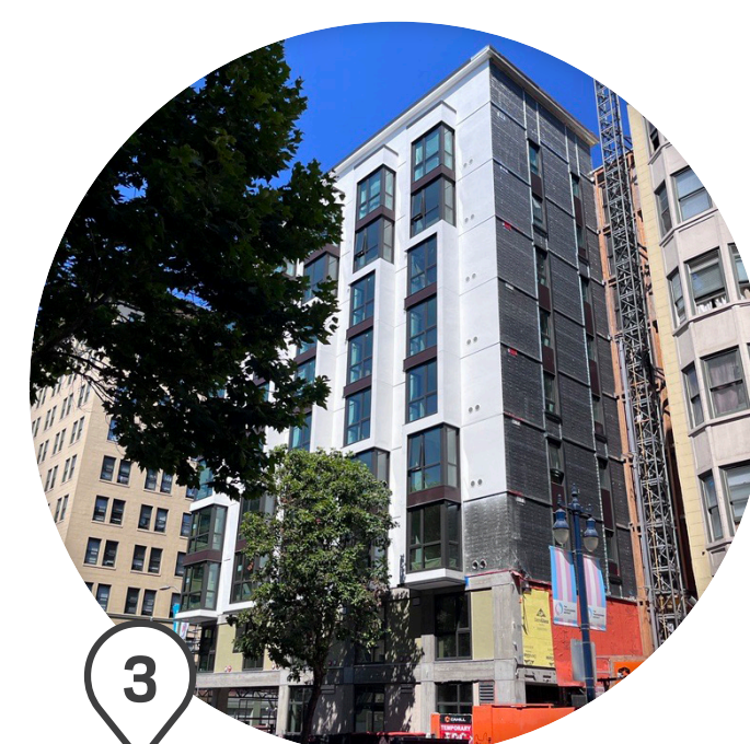
180 Jones St. (New Affordable Units)
