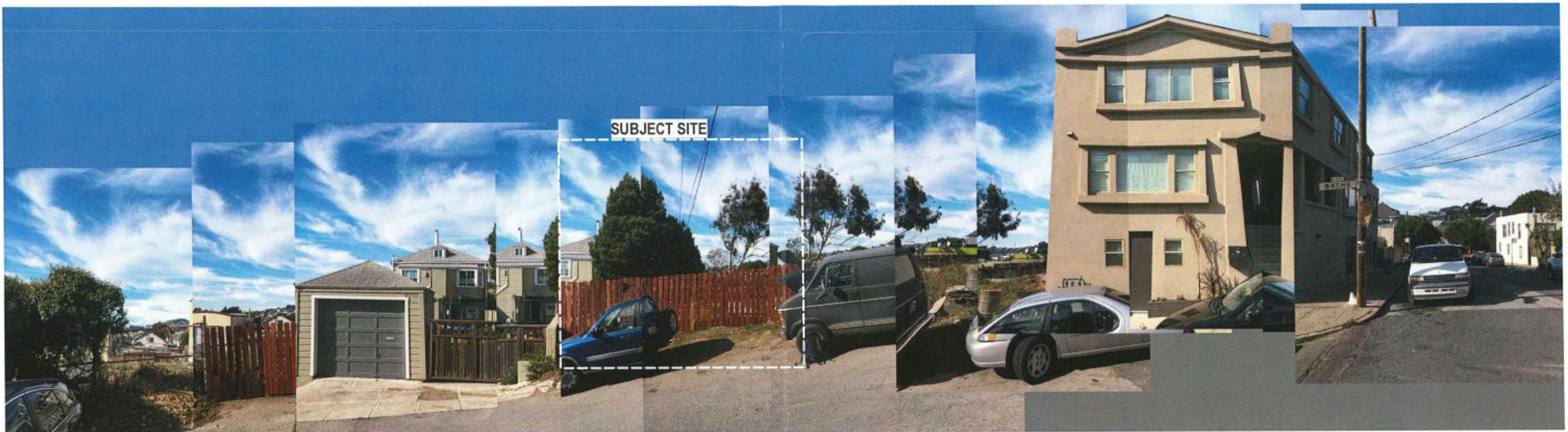
SUBJECT AND ADJACENT BUILDINGS ON BACHE STREET (LOOKING WEST)
