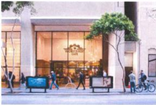
Workshop's street LEVEL RETAIL presence from Montgomery St
